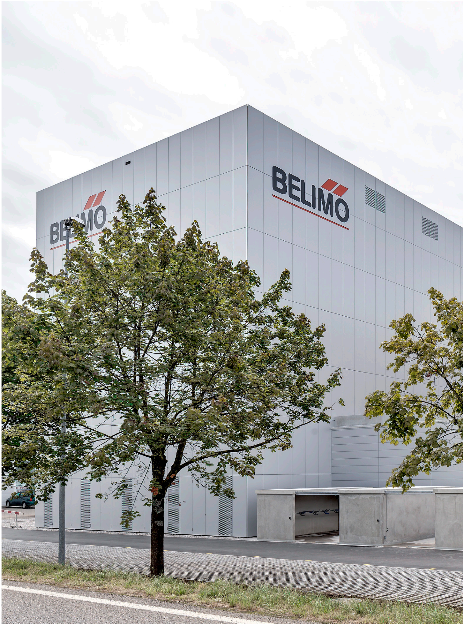
Expansion Building high-bay warehouse
