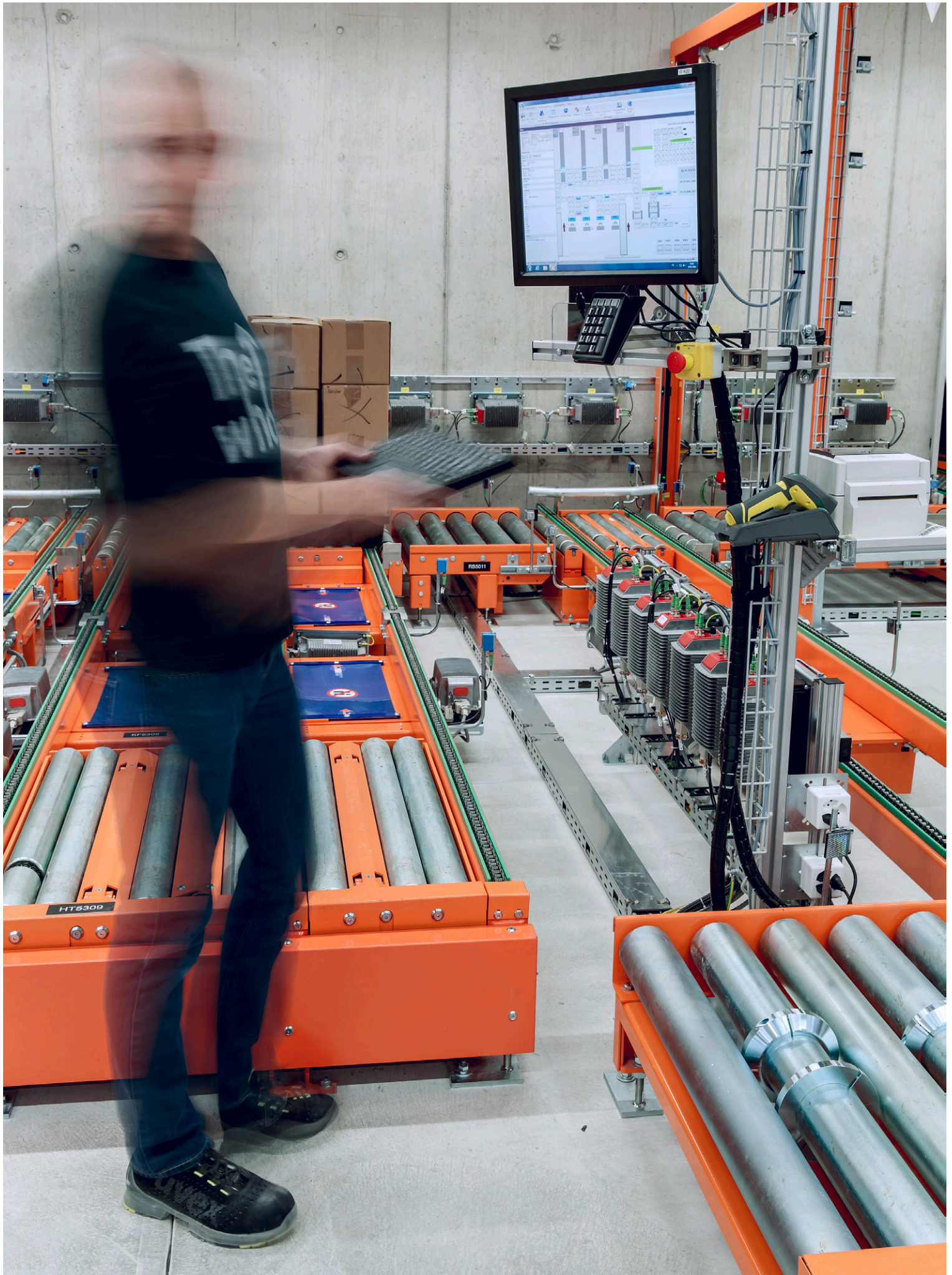
Picking-area high-bay warehouse
