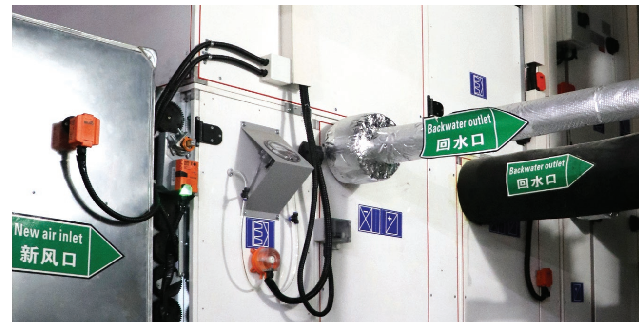
Belimo provides a complete range of innovative HVAC field devices for AHU applications.
