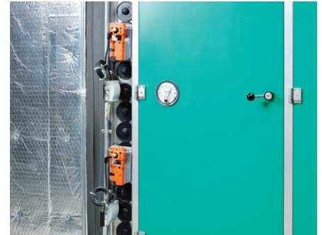
Damper actuators on air handling unit
