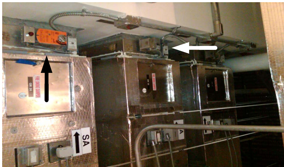
Typical replacement – white arrow shows location of Honeywell and black arrow shows replacement Belimo.
