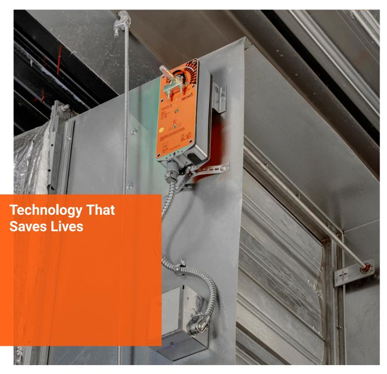
**Fire and Smoke Damper Actuators**
