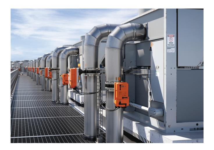
Butterfly Valves are fundamental components in hydronic systems. Unfortunately, most butterfly valves are less than ideal – they leak, their running times are not optimized for HVAC applications, they're heavy, it's hard to access wiring, and they cannot be put into operation quickly.
