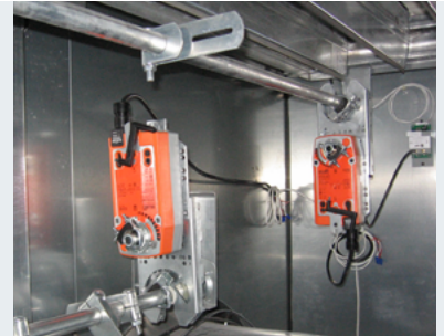
AIR HANDLER DAMPER ACTUATORS 22...1400 in-lb
